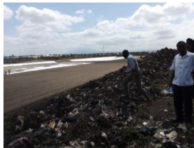
SLF under construction in Arusha, Tanzania
